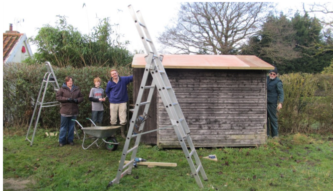
Clare & John of the Village Hall Committee with extra help from Rob & Jack repairing the Village Hall Hut.
