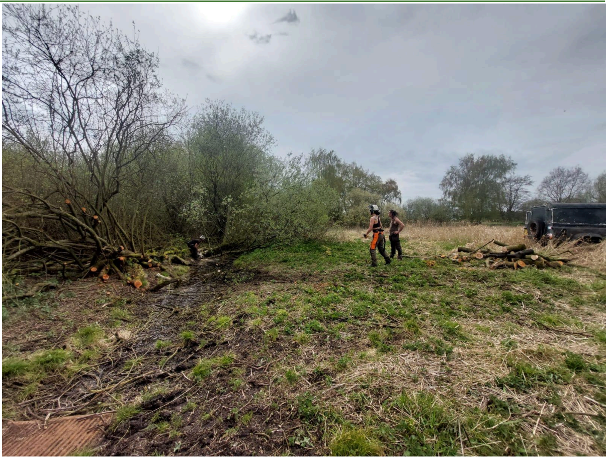
Tree work and land clearance on the iFarm site – volunteers hard at work
