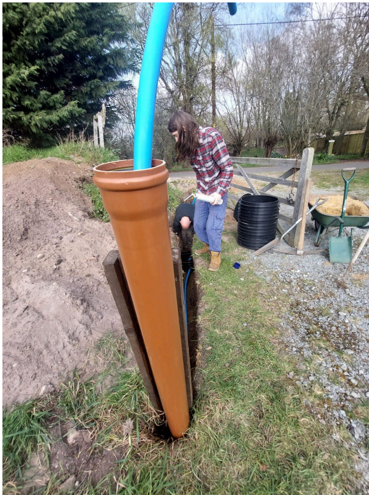
Standpipe installation in progress, March/April 2026 – connecting the mains supply to the farm site
